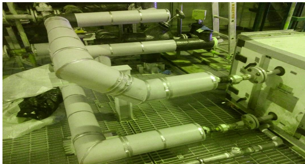
Chiller Water Piping Installed at B-03 KFU site – Al Hasa
