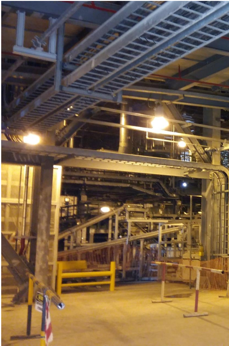
Electrical Cable Tray Installations
