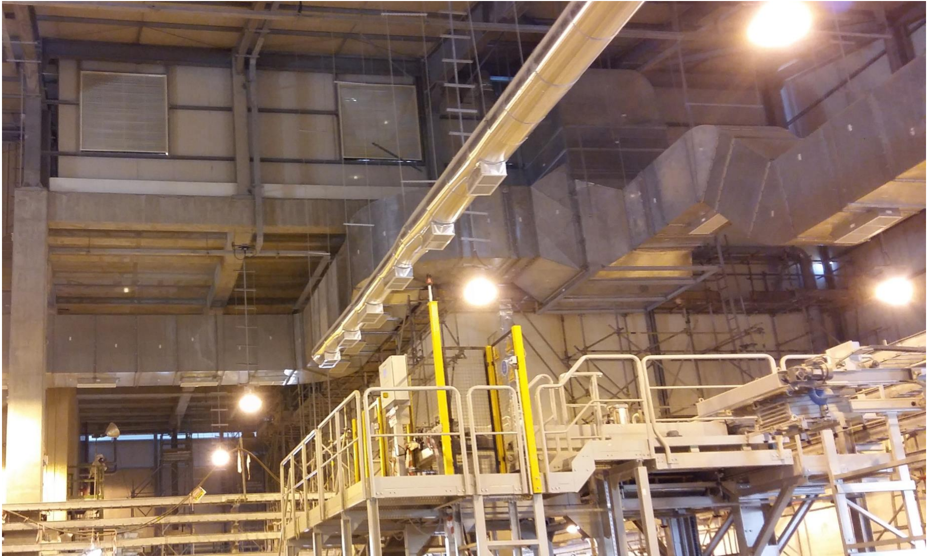
Air Louvers & Ductworks Installed at High Levels
