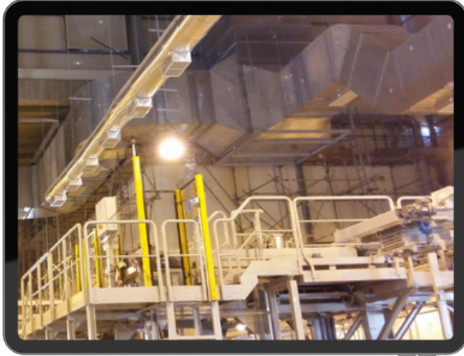
HVAC DUCTS INSTALLED AT HIGH LEVELS AT KEMYA SITE
