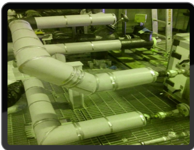
CHILLER WATER PIPING INSTALLED AT B-03 KFU SITE – AL HASA
