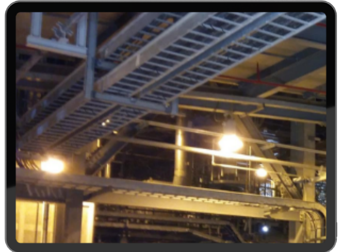
ELECTRICAL CABLE TRAY INSTALLED AT KEMYA SITE
