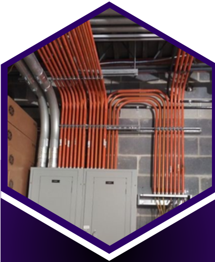
Installation of PVC/EMT/RGS conduit (embedded/exposed) and all relevant accessories
